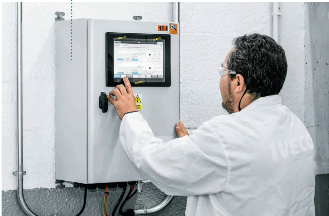
The compact design of the energy efficiency module means that it fits in the ATEX safety cabinet. It is operated using a touch screen, smartphone or tablet.
