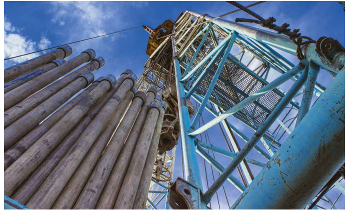
Geological bore drilling
