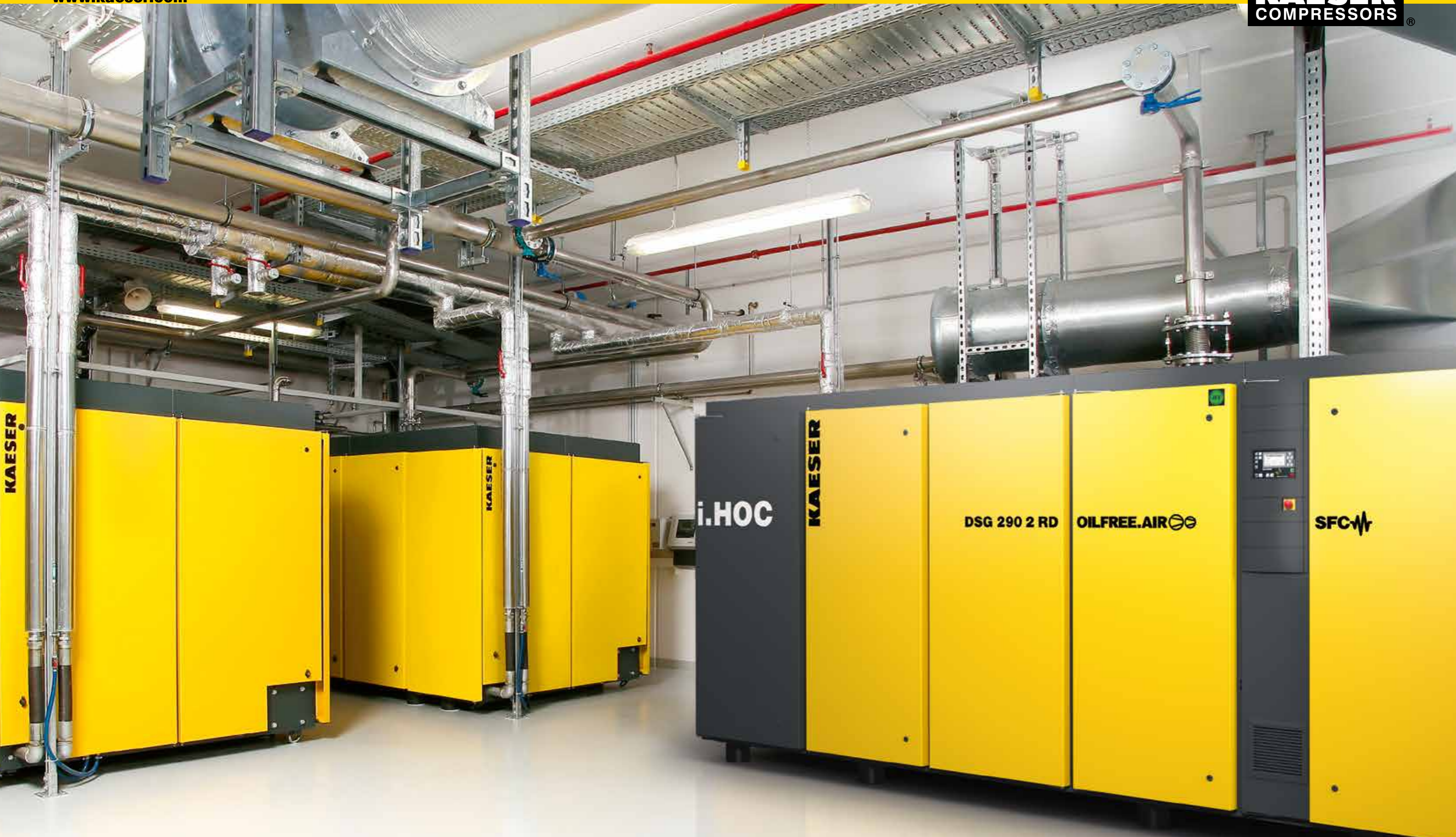
Image: Example of a KAESER station that has been expanded with the installation of a water-cooled DSG 290-2 RD SFC dry-running rotary screw compressor.
